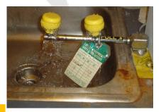
Remember: These devices are in place for your protection. Monthly flushes keep sediment and debris from accumulating in the lines which could potentially cause harm to your eyes in case of emergency use!!
